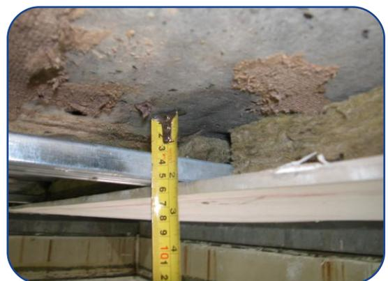
CB-RR-50 with C Channel, fibreglass and gypsum board
