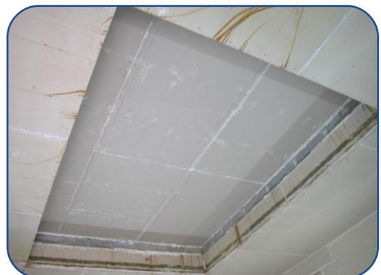
Finish the installation of gypsum board and sealant
